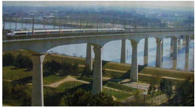
Trains like the 220 MPH TGV in France must have their own dedicated infrastructure like this multi-million dollar bridge built new in order to safely reach their top speeds.
